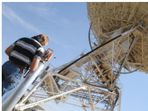
Fig. 2 Ludwig Combrinck surveying the 26m's polar shaft during bearing repair (Credit: Mike Gaylard).
